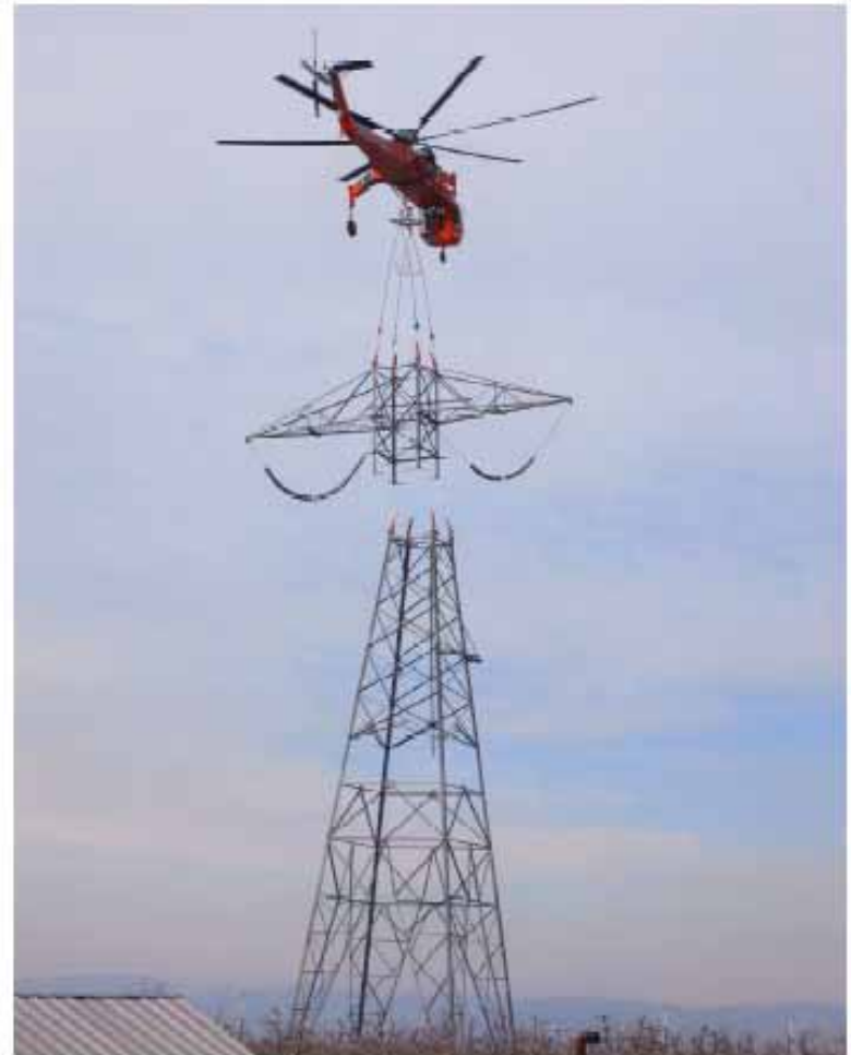
Helicopter sets tower top for the new Schultz-Wautoma 500-kV transmission line.
